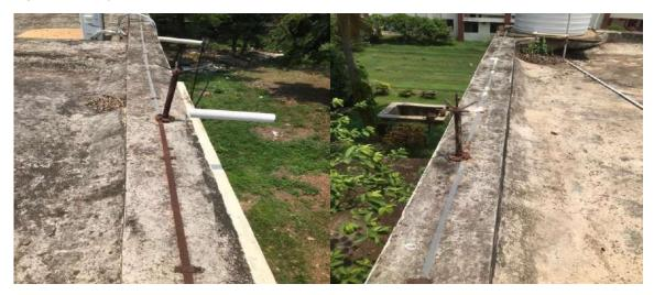
Fig. 50 – Lightning Arrestors in the Terrace of Institute's Main Building and D.M.School Building
